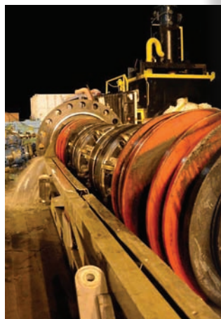
Below TDW's SmartPlug tool emerges from temporary launcher
